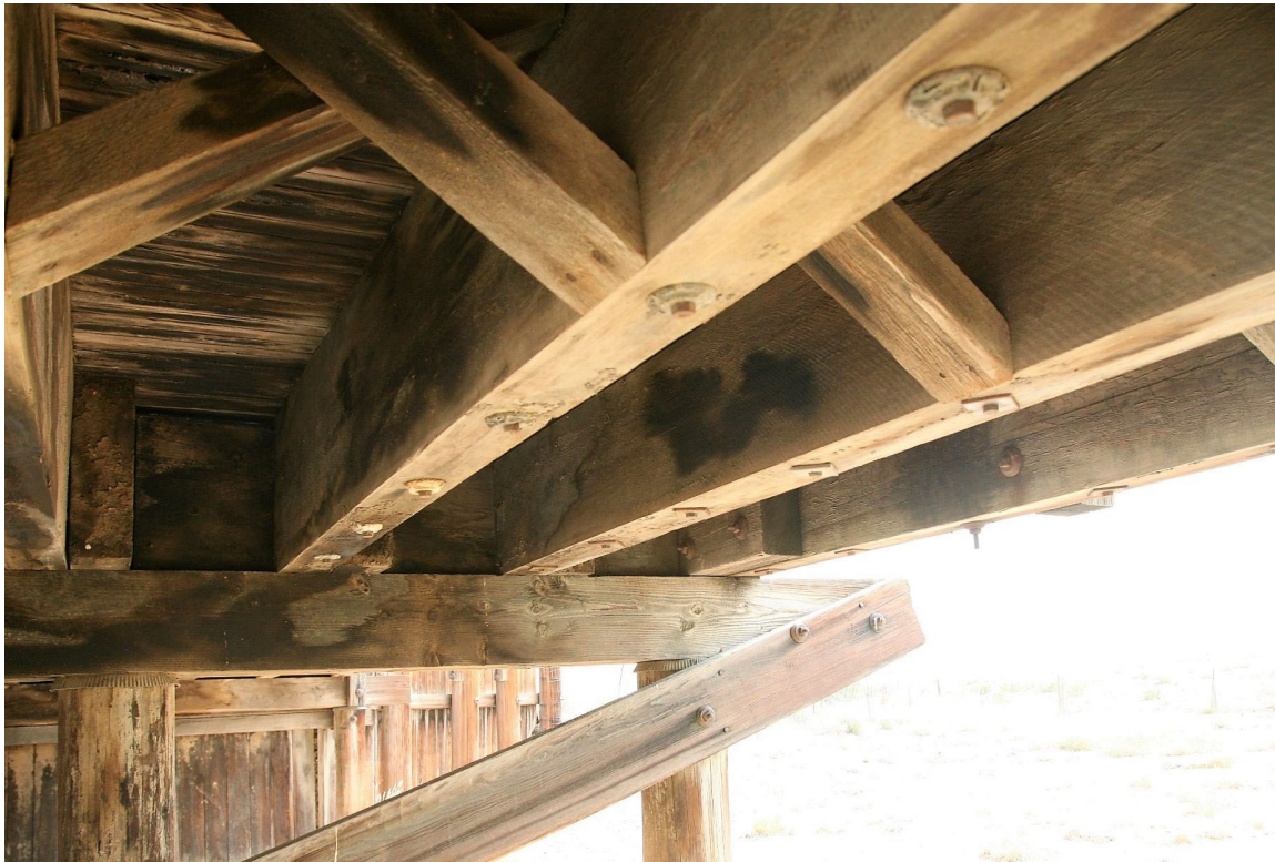
Picture 2 - Repaired Girders
