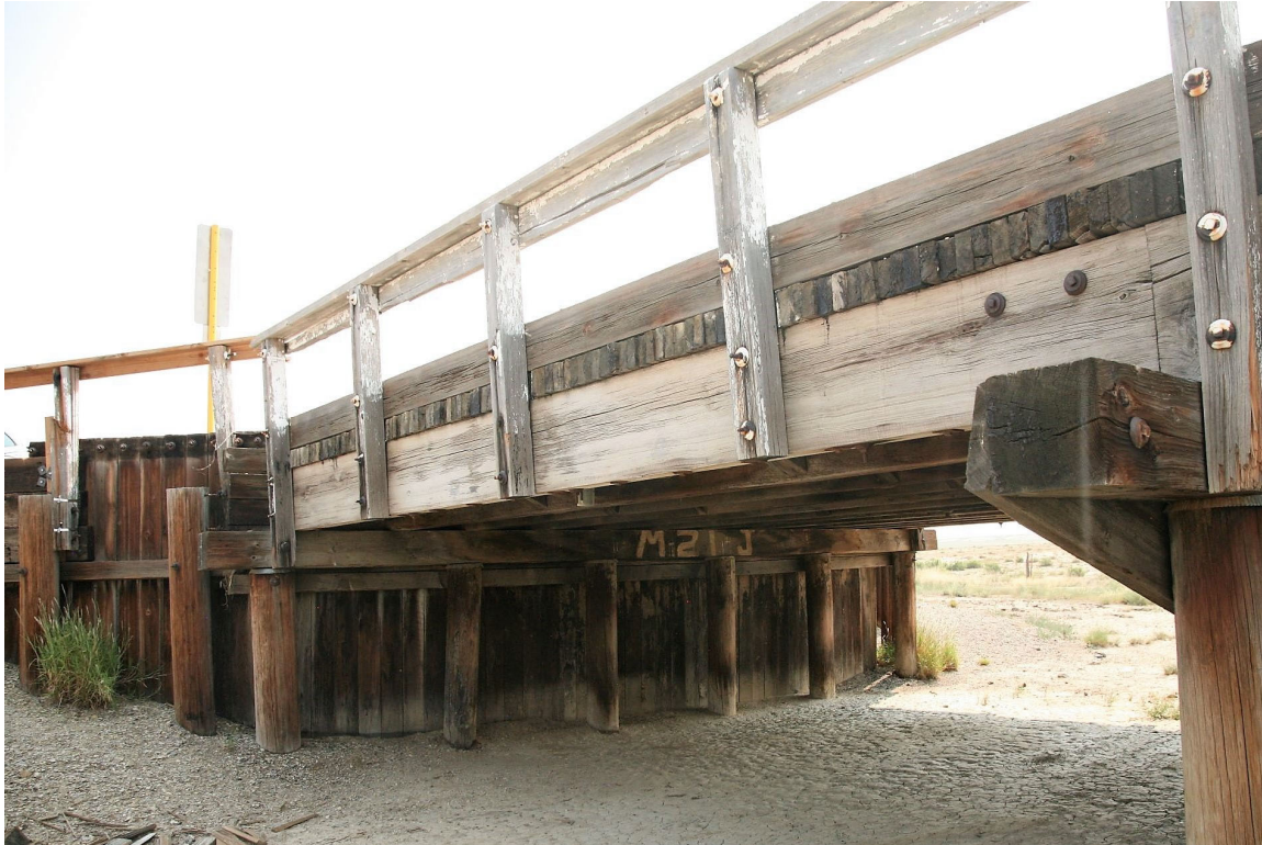
Picture 3 - Girders, Guardrail, Piles
