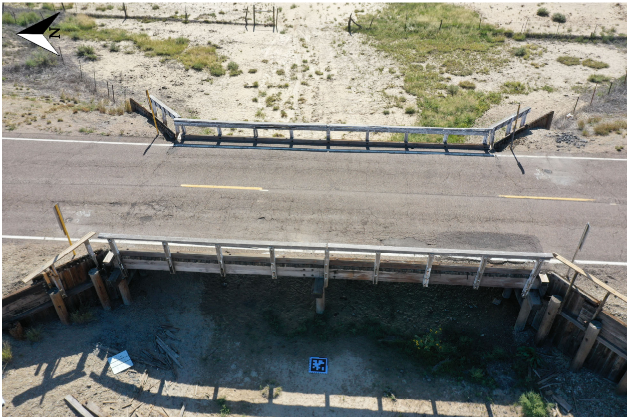
Picture 1 - Bridge M-21-J
